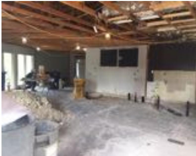
Speaking of safety, everyone on site needed ear protection early in the week with lots of jack hammering and cement saws. All the tile in the entrance way has been removed and they have cut through the foundation to access the sewer lines. As you can see in the photos, all the supporting plumbing for the bathrooms is now complete.
